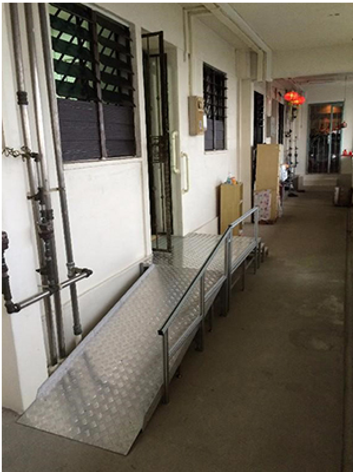
Customised ramp, suitable for units located along the corridor
