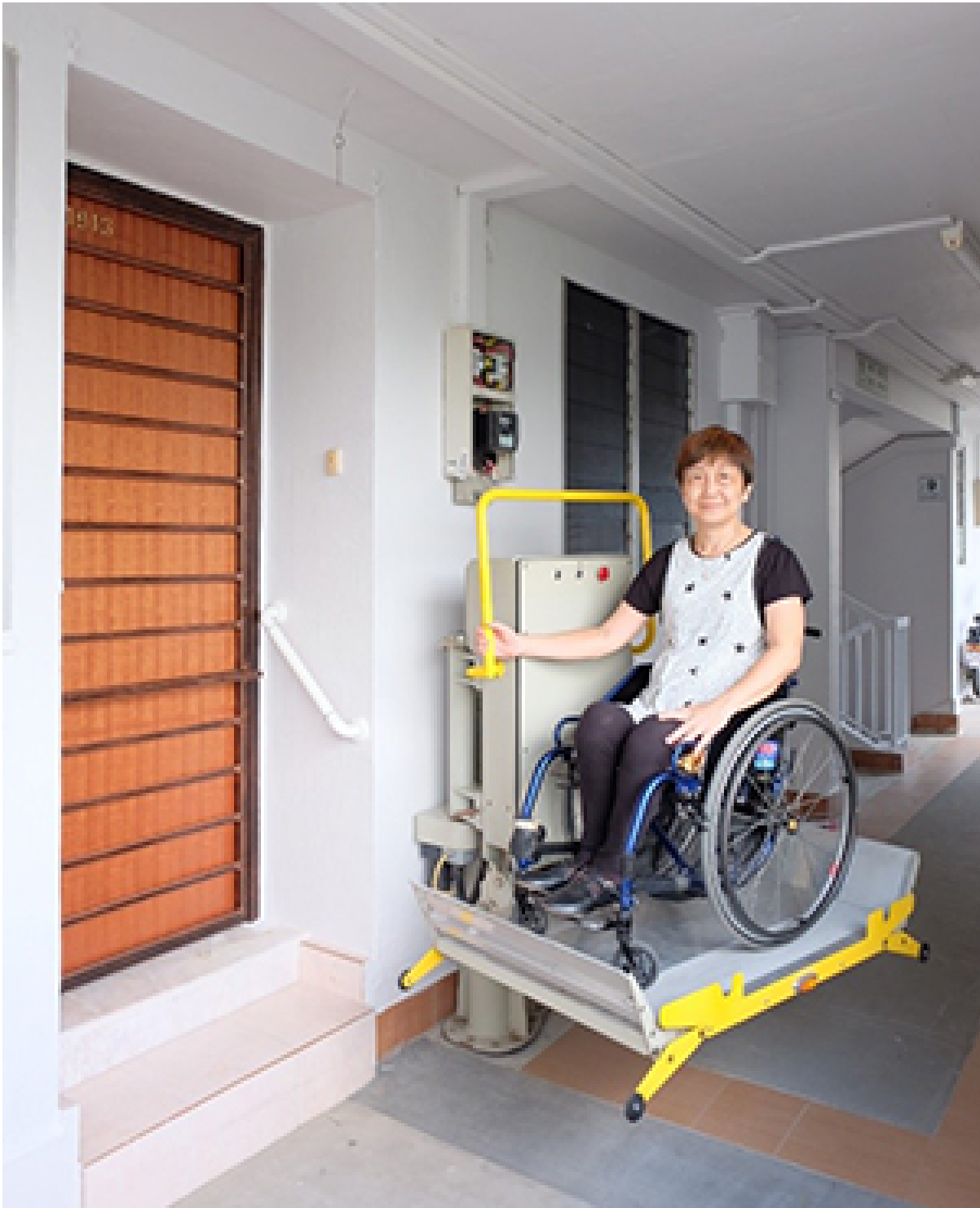
Wheelchair lifter, for units with site constraints
