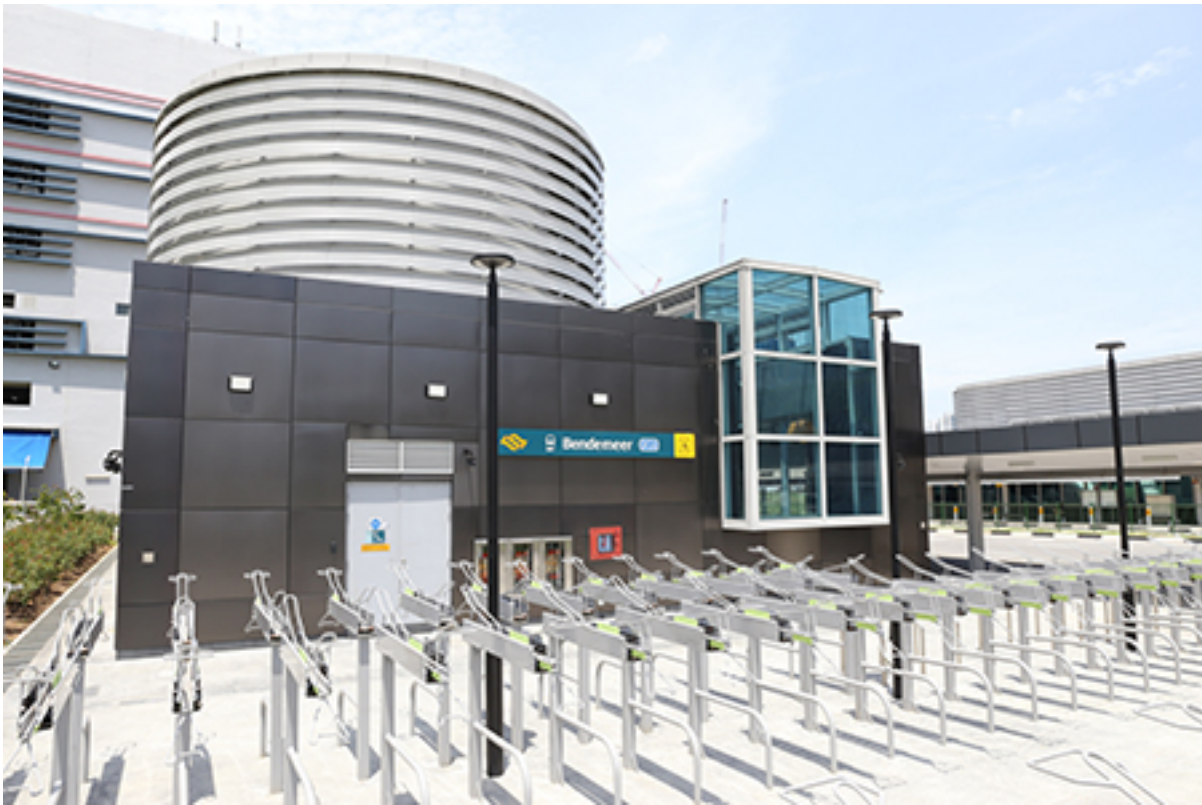
Bicycle parking lots at Bendemeer Station
