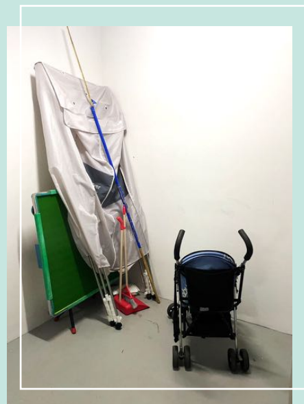
An example of stairwell cluttering witnessed at Goodview Garden
