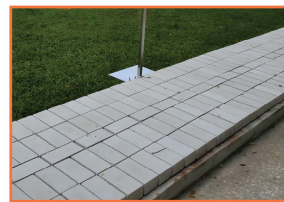
Trial casting using MgO cement e.g. pavement blocks
