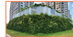
GBS - sustainable retaining structure
