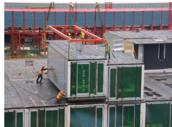
Prefabricated prefinished volumetric construction (PPVC) for student hostel @NTU
