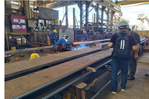
Fabrication of the 1 st S690 King Post in SG
