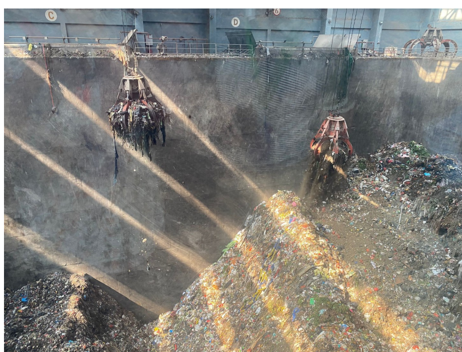
The Integrated Waste Management Facility and Tuas WRP form the Tuas Nexus.
