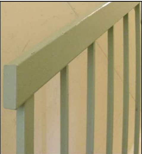
Staircase railings in good condition
