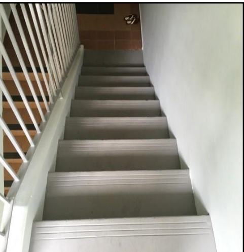
Staircase in its clean state
