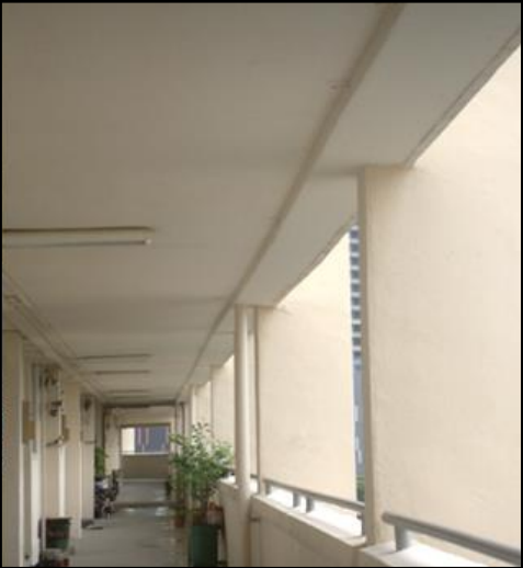
Corridor without any unauthorised structure
