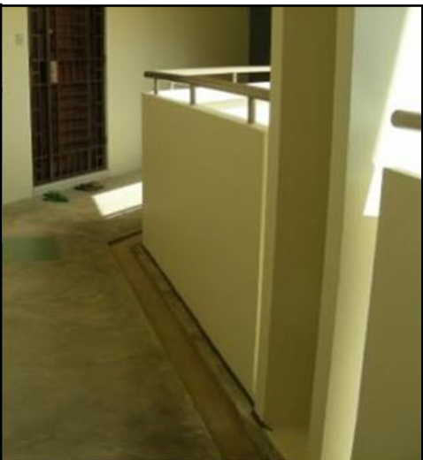
Corridor free from obstruction
