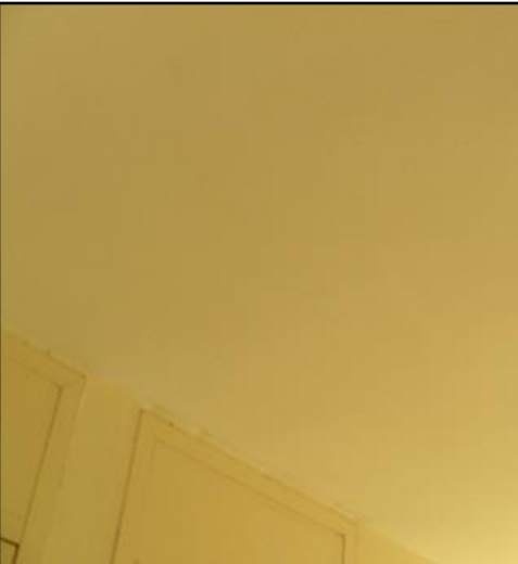
Corridor ceiling in good condition
