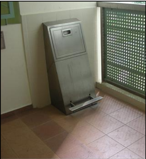
Central refuse chute area free of dumping
