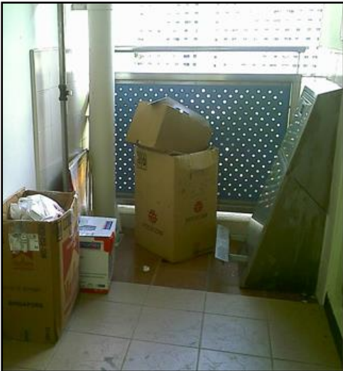
Central refuse chute area dumped with refuse
