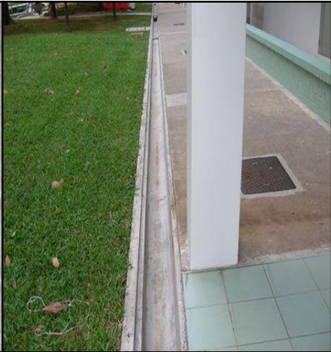
Apron drain free from litter
