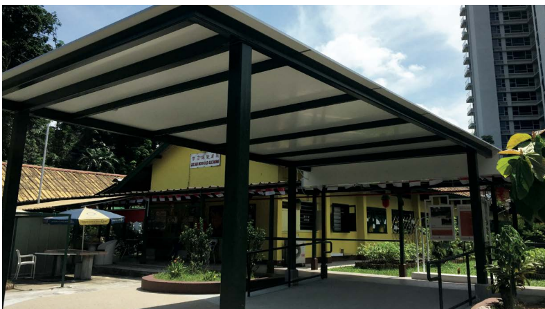
A new sheltered drop off point for ambulances and other vehicles to transport residents more easily, rain or shine.
