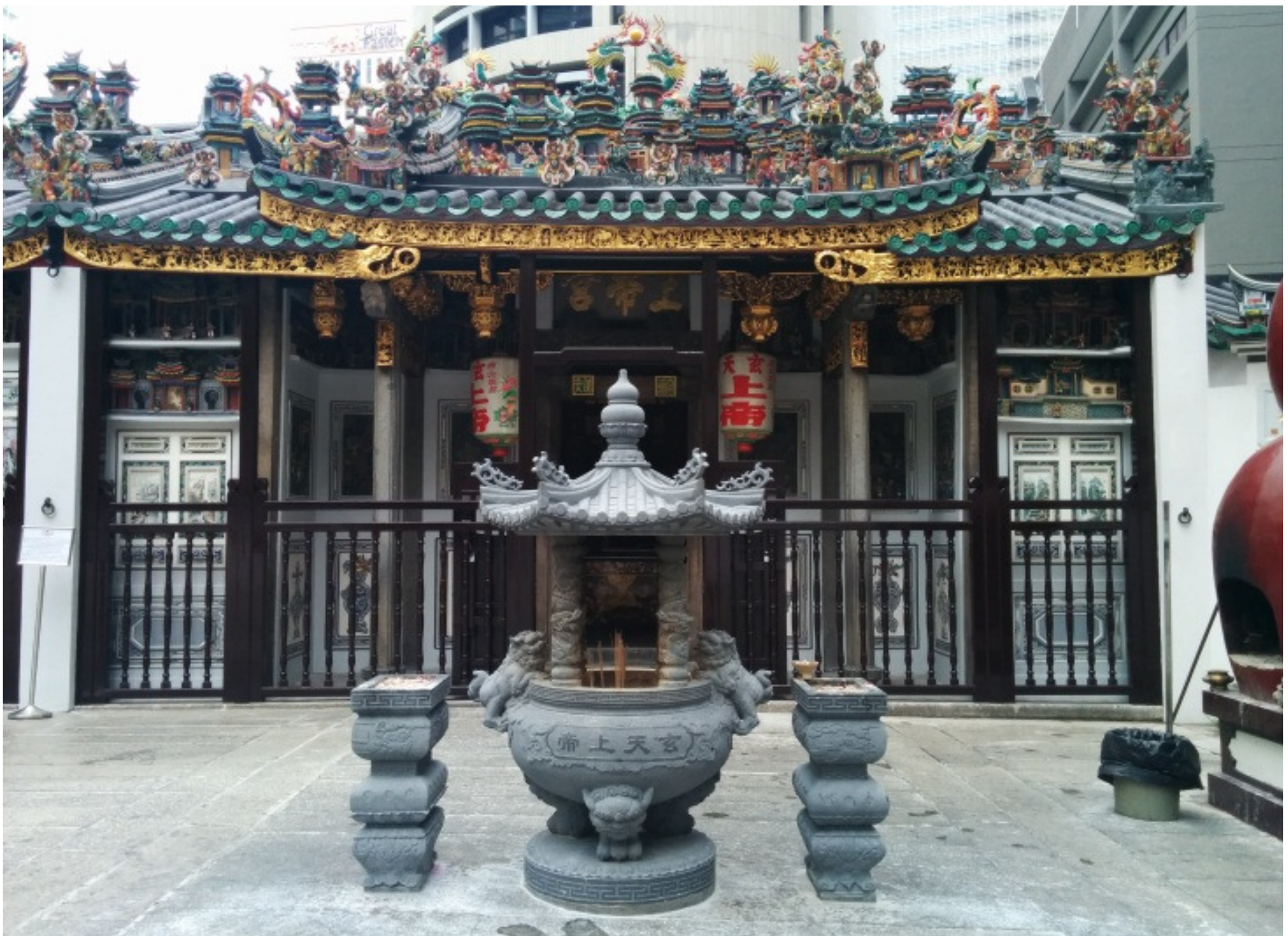
Yueh Hai Ching temple after restoration works
