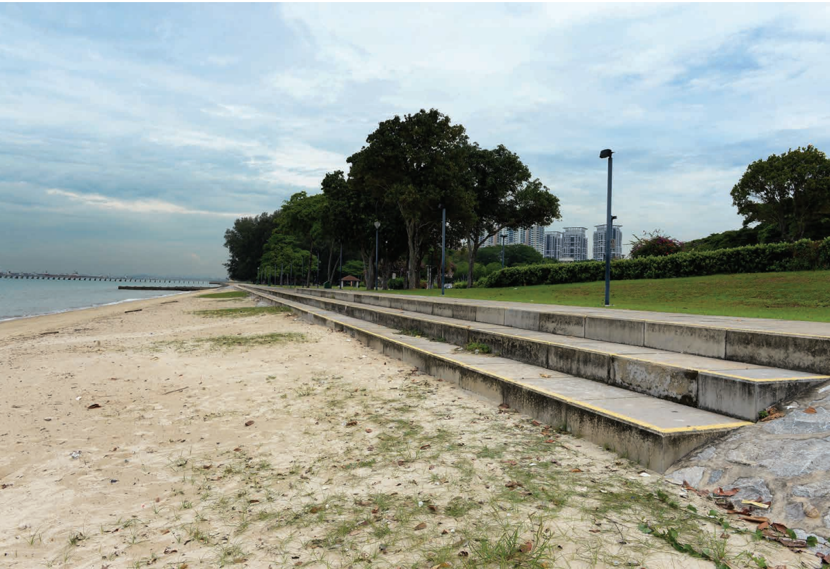
Composite stepped seawall at East Coast Park
