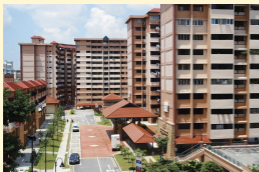
The first upgrading programme at Ang Mo Kio Ave 3 was announced in 1990 and completed in 1995.
