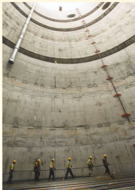
Inside the Deep Tunnel Sewerage System.
