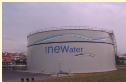
Tank at the Bedok NEWater factory, taken at the official launch of NEWater and the opening of the NEWater Visitor Centre, 2003. Photo credit: Ministry of Information, Communications and the Arts Collection, courtesy of National Archives of Singapore
