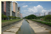
The concrete canal in Bishan Park before it was naturalised under the ABC Waters Programme. Photo credit: PUB
