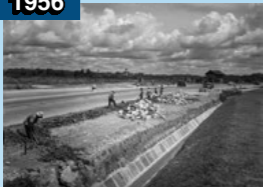
Road construction in a rural area, 1956.
