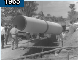
Laying water pipes, 1965.
