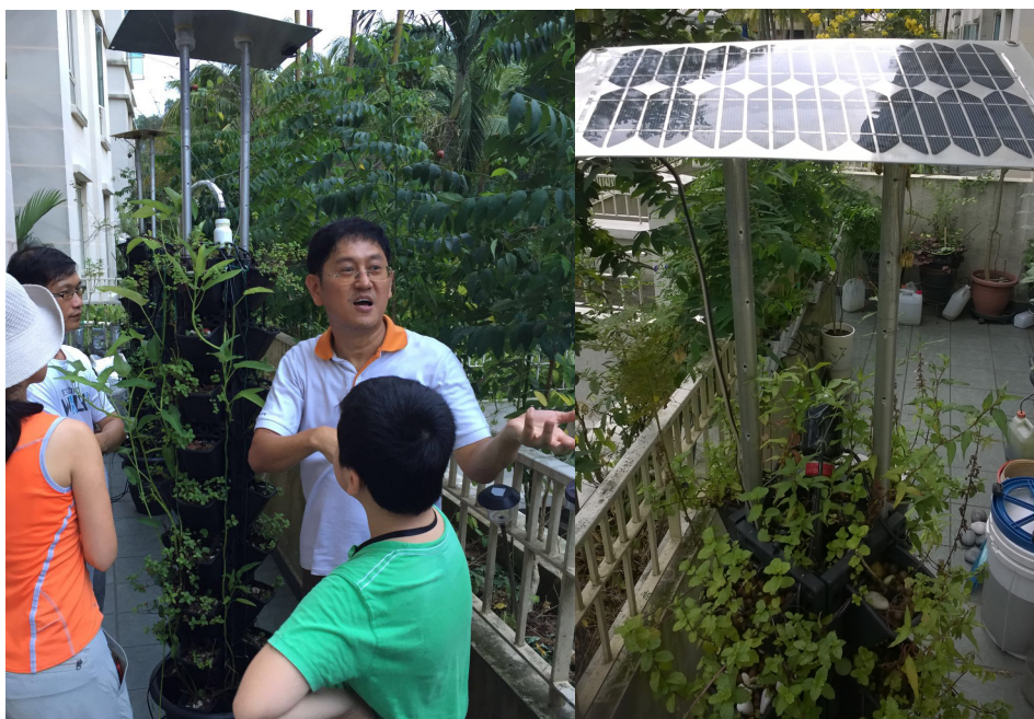
(Left) Ben explaining the solar-powered vertical aquaponics system in his garden. (Right) Solar panels help to power the system.
